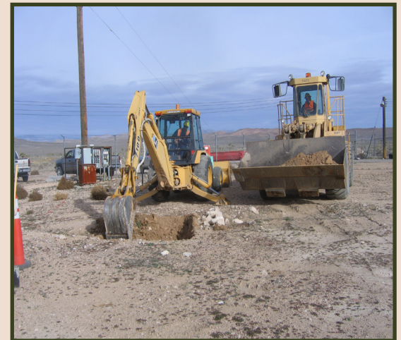
Sample collection with a backhoe at a Complex Process site on the Nevada National Security Site
