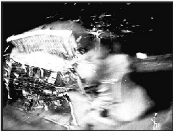
"Annie" a 16-kiloton atmospheric test fired from a tower on March 17, 1953, destroyed this house in less than three seconds.
