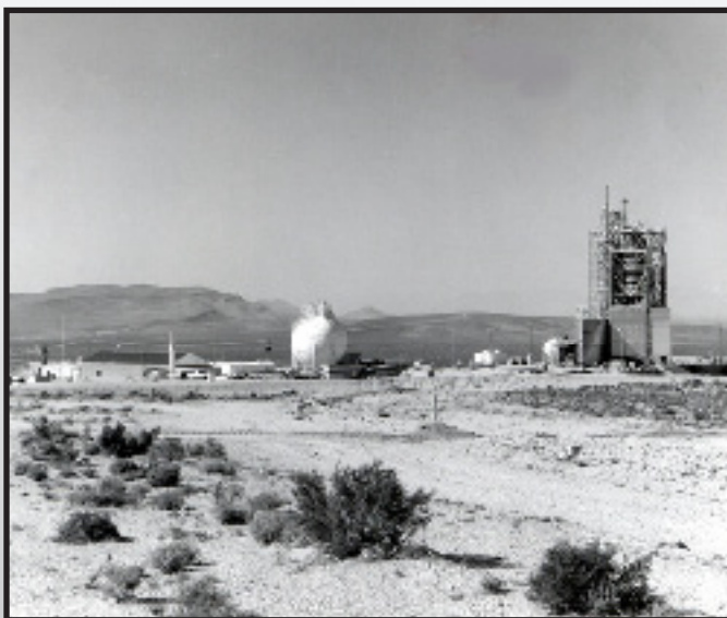
Liquid hydrogen tanks at the Nuclear Rocket Development Station.
