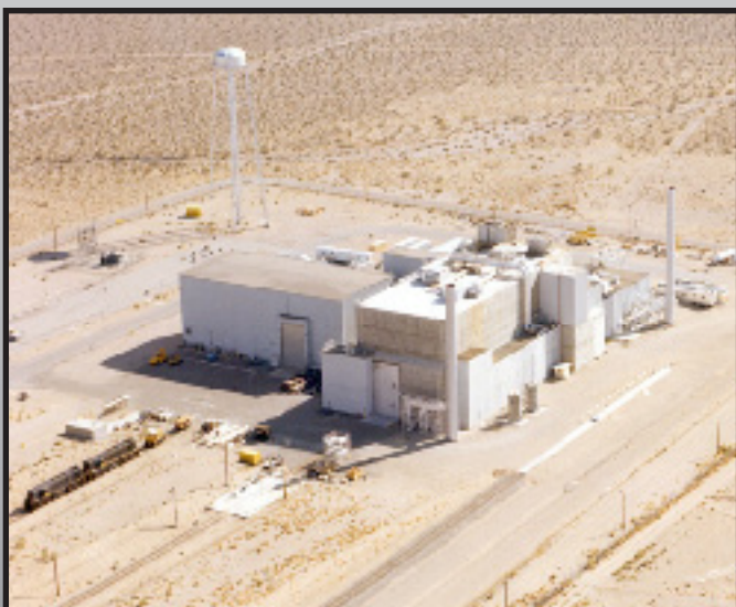
The E-MAD building contained a state-of-the-art hot bay, six-foot thick walls, and a 32-inch thick roof.
