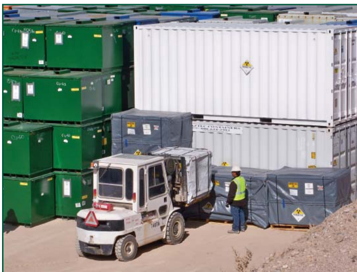
Packages of low-level radioactive waste are positioned in a disposal cell at the Area 5 Radioactive Waste Management Site.
