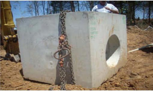
Victim was in an excavated ditch. A concrete box was being lowered into the ditch when the rigging broke and the box fell on him.
