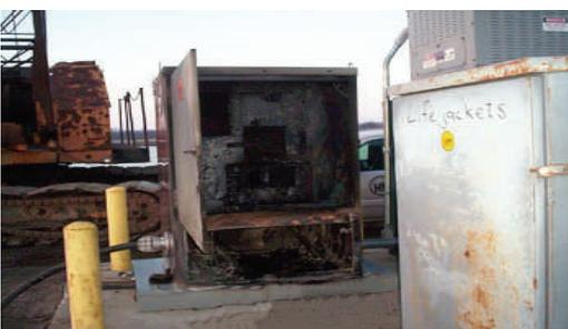
Victim was attempting to connect a 4160 volt cable from the dredge to the load side terminals in electrical panel when he contacted energized terminals.
