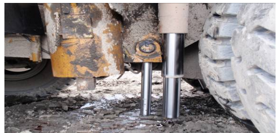
Hoist Cylinder Failure
