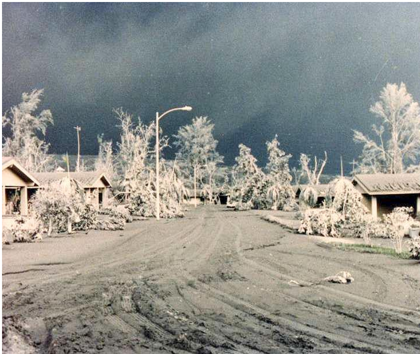
Figure 6: Base housing at Clark AB covered with ash after the eruption. Many buildings' roofs collapsed under the weight of the ash.
