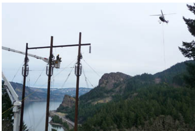
Crews install a new wooden structure on the Bonneville-Hood River line.
