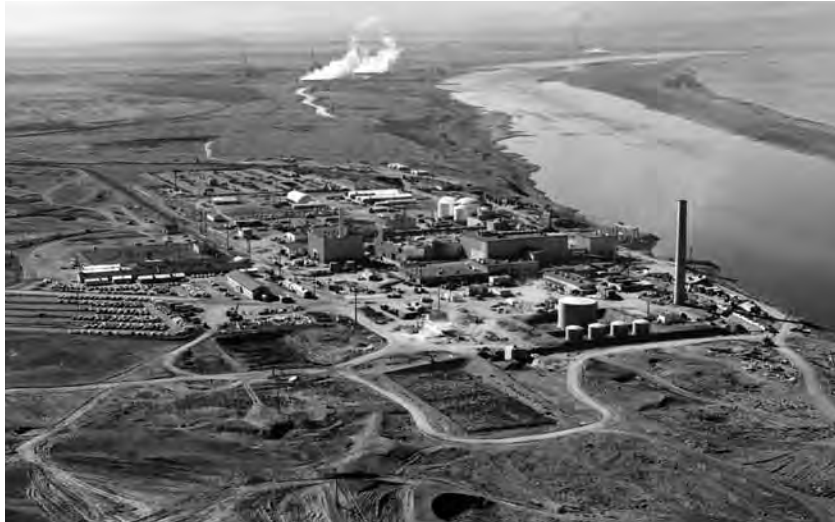
Hanford's N Reactor is called a dual-purpose reactor because it not only produced plutonium for America's defense program, but also generated electricity marketed by BPA. At construction in the early 1960s, it was the only reactor of its kind in the nation.
