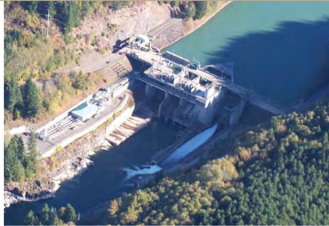
As part of BPA's Resource Program, the agency acquired the output of the 70-megawatt hydroelectric development at the Cowlitz Falls Dam, owned and operated by the Lewis County Public Utility District.
