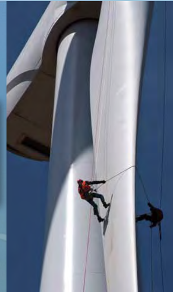
A worker scales a massive blade that drives a modern wind turbine’s power generator. The advent of wind farms in the Northwest has created high-tech jobs and stimulated local economies.
