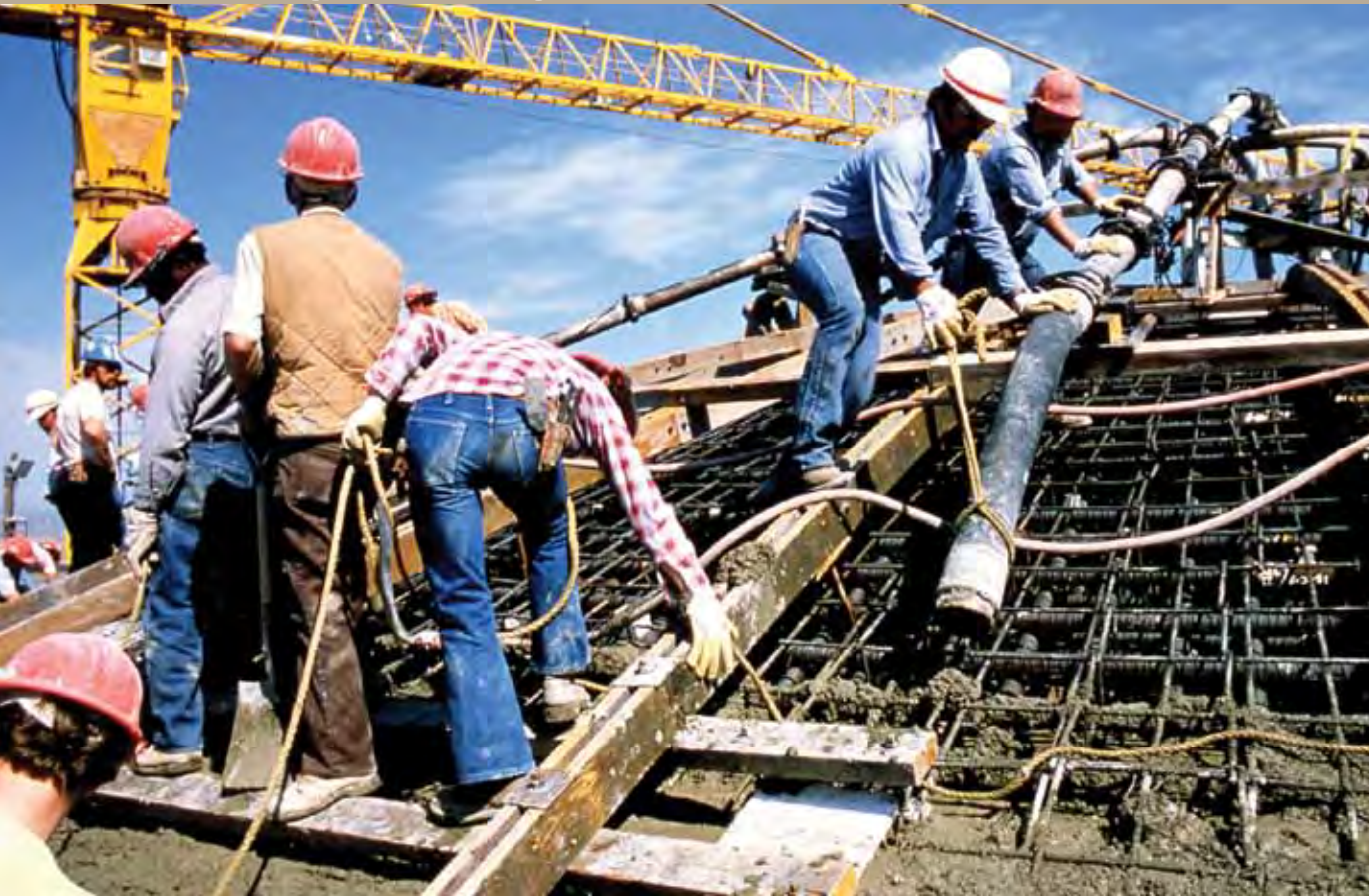
Workers pour concrete for the containment dome at WNP-2. Now known as the Columbia Generating Station, it was the only nuclear plant completed. Energy Northwest (formerly WPPSS) owns and operates the plant and BPA purchases and markets its output.
