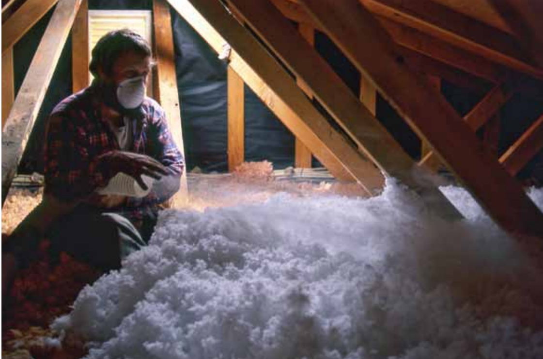
Home weatherization was a flagship of the first suite of BPA conservation programs. Contractors retrofitted insulation in the attics, walls and crawlspaces of electrically heated homes to reduce their energy usage.
