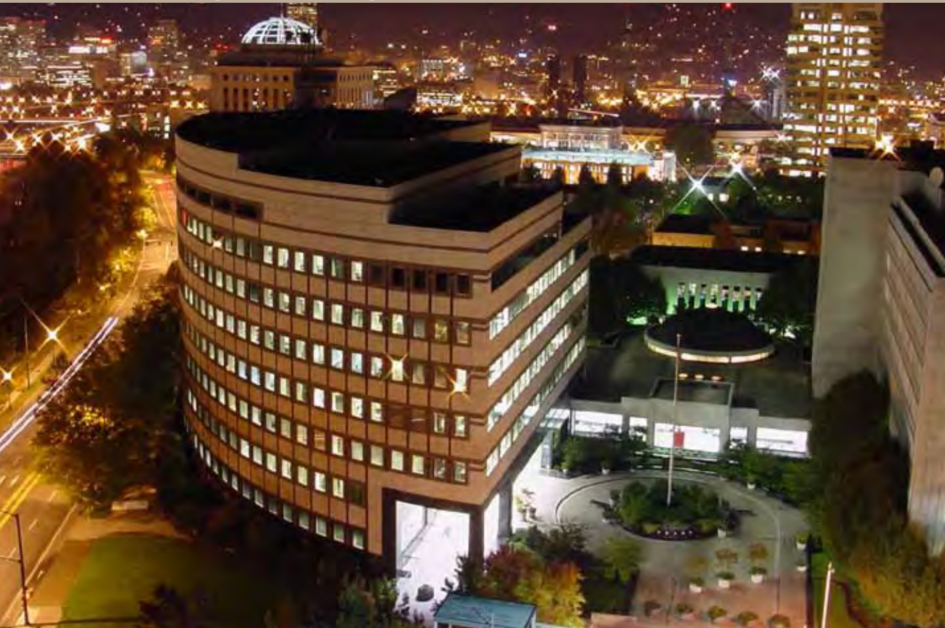
BPA's headquarters building in northeast Portland houses about one-third of the agency's workforce.
