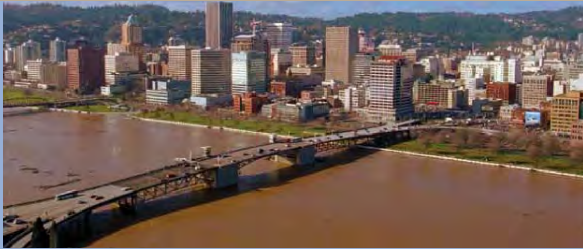
Coordinated management of federal dams on the Columbia and Willamette rivers kept the Willamette inches from topping the seawall in downtown Portland, Ore., during the flood of 1996. Locals piled sandbags along the seawall to keep the water back. (AP Photo/Jack Smith)
