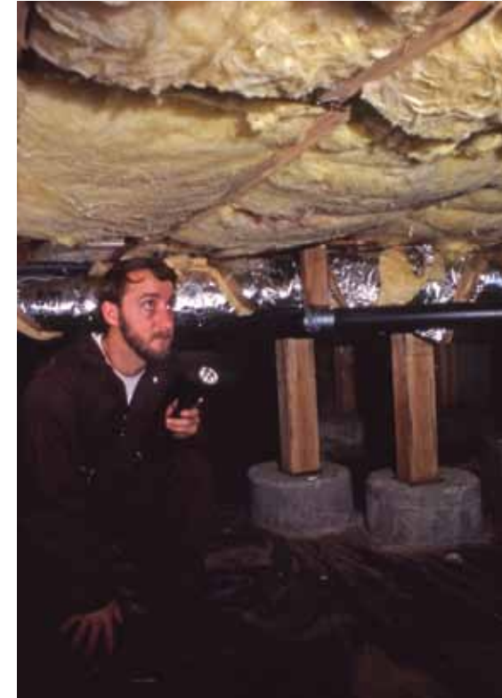
BPA engineers peered into crawlspaces to inspect insulation jobs for the weatherization program.
