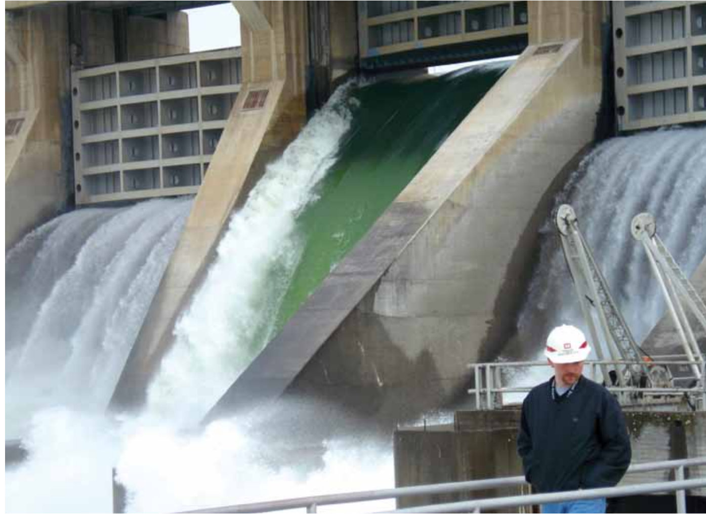
Water rushes over a spillway weir at McNary Dam, easing the downstream migration for juvenile salmon and steelhead by providing passage at the river’s surface — where they naturally migrate. (Scott Bettin/BPA)
