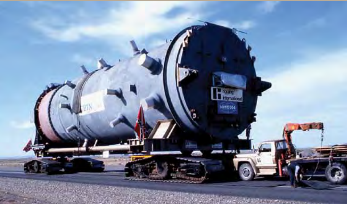
A nuclear reactor vessel slowly crawls toward WNP-2, now the Columbia Generating Station, during construction in April 1976. The vessel holds nuclear fuel rods that drive the nuclear reaction to produce energy.
