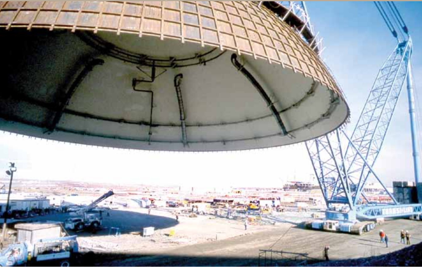
Work begins on Washington Nuclear Plant 1, developed by the Washington Public Power Supply System with financial backing from BPA.
