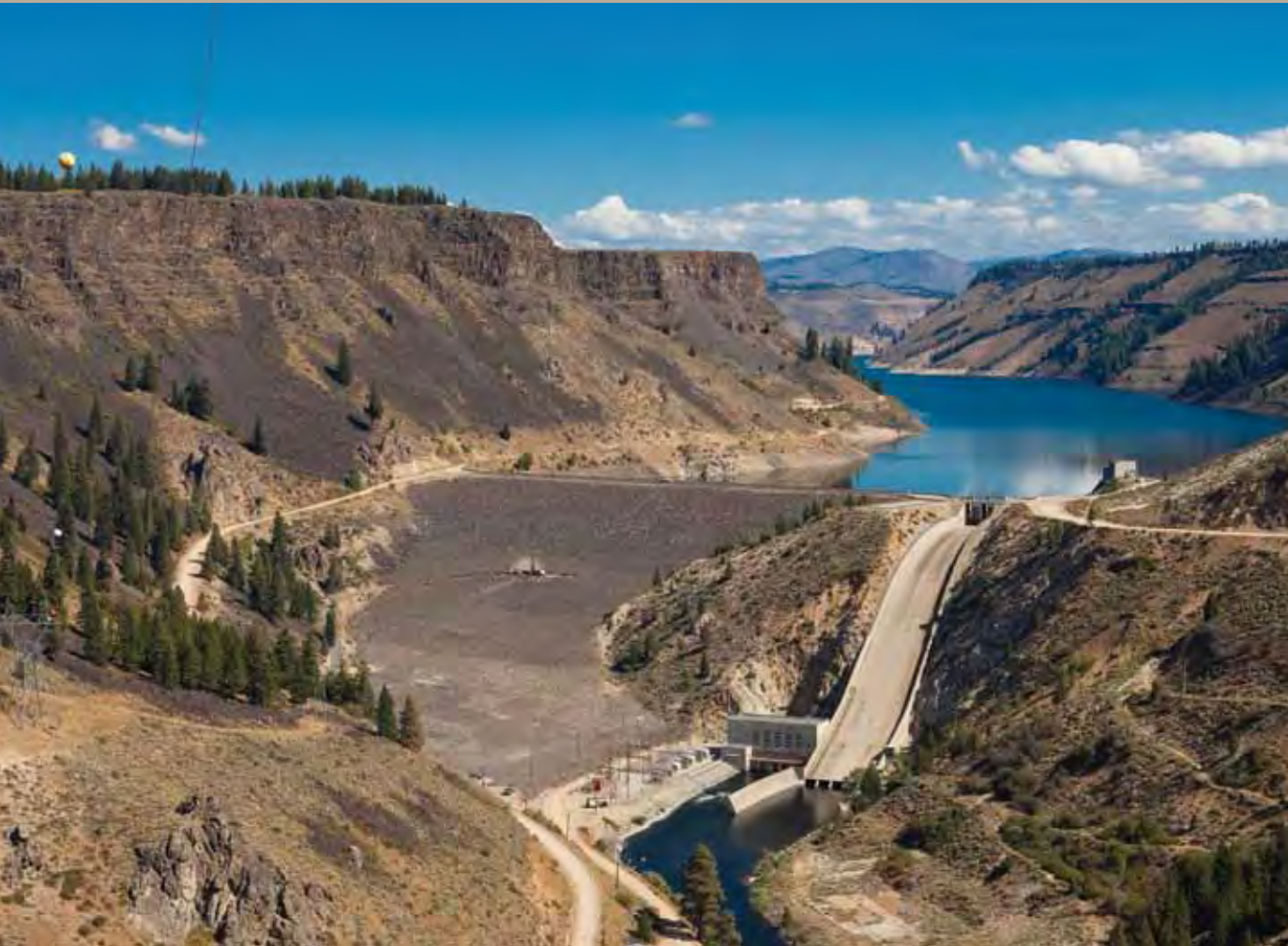
Anderson Ranch Dam on the South Fork of the Boise River north of Mountain Home, Idaho, is one of the smaller dams in the federal system. Its two generating units were updated in 1986 to a combined capacity of 40 megawatts.
