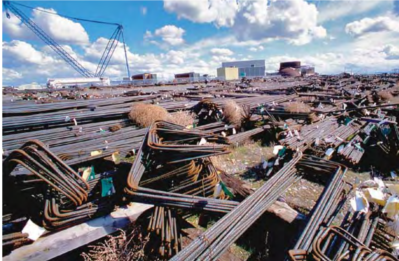
Building materials at the idled construction site of WNP-4 in 1982.
