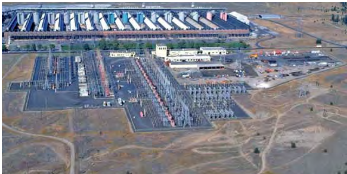
Kaiser Aluminum plant near Spokane, Wash., with BPA's Bell Substation in the foreground.
