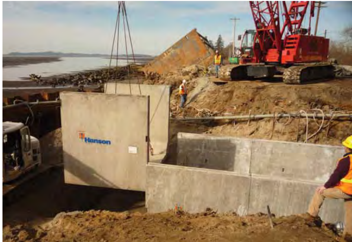
Workers install a large culvert to reopen historic wetlands in the Columbia River estuary to provide food and refuge for juvenile salmon and steelhead. The young fish build strength in the estuary before setting out into the ocean. (David Wilson/BPA)
