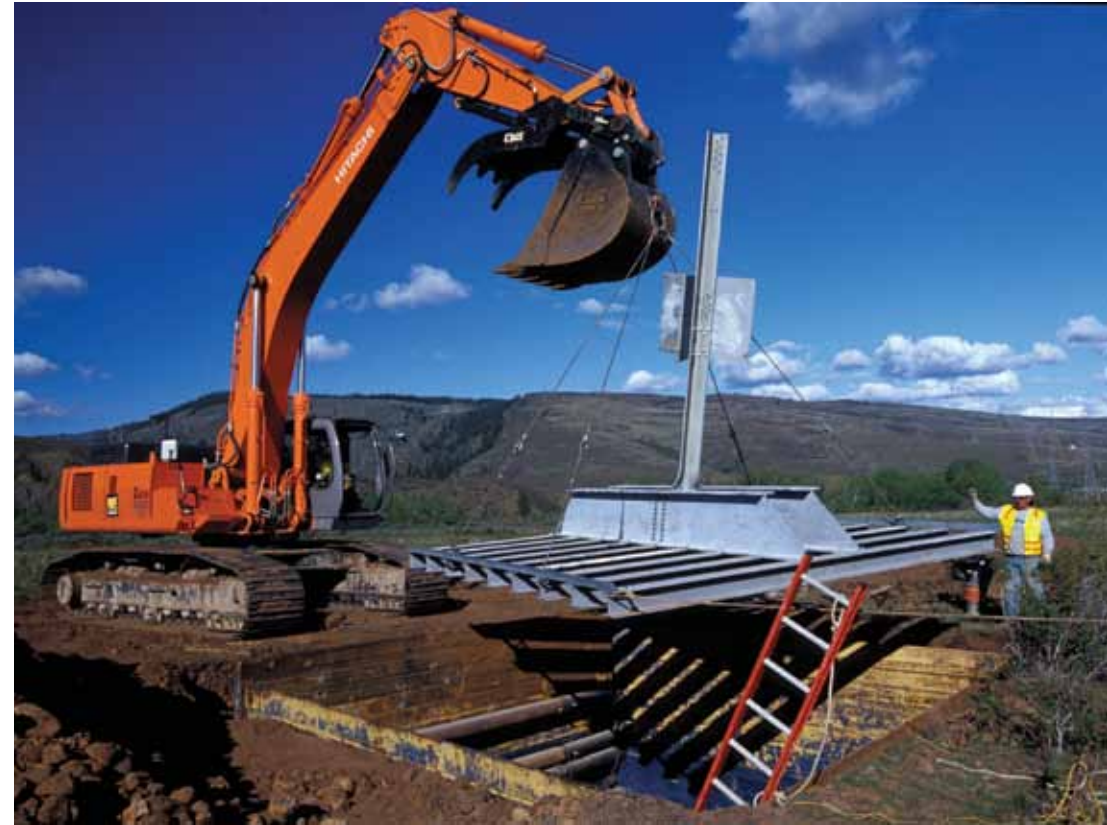
Crews install a transmission tower footing during construction of BPA's Schultz-Wautoma line.
