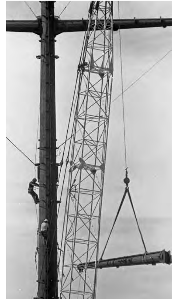
A crane lifts a section of a 175-foot single-shaft transmission tower.
