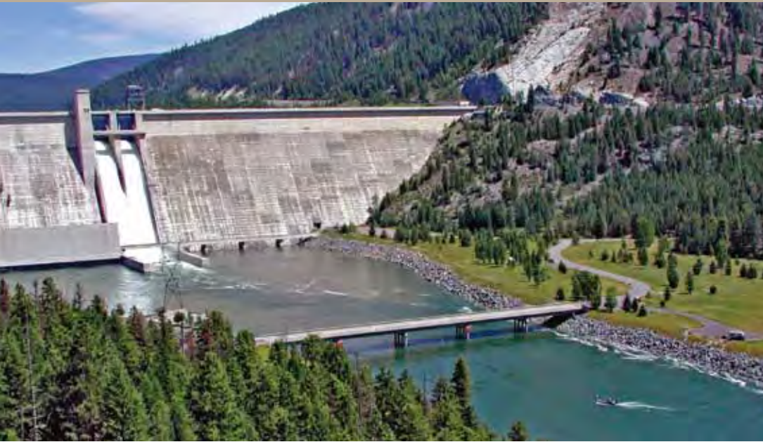
Libby Dam in northwest Montana was the fourth and final dam built under the Columbia River Treaty, and is the only treaty dam in the United States.
