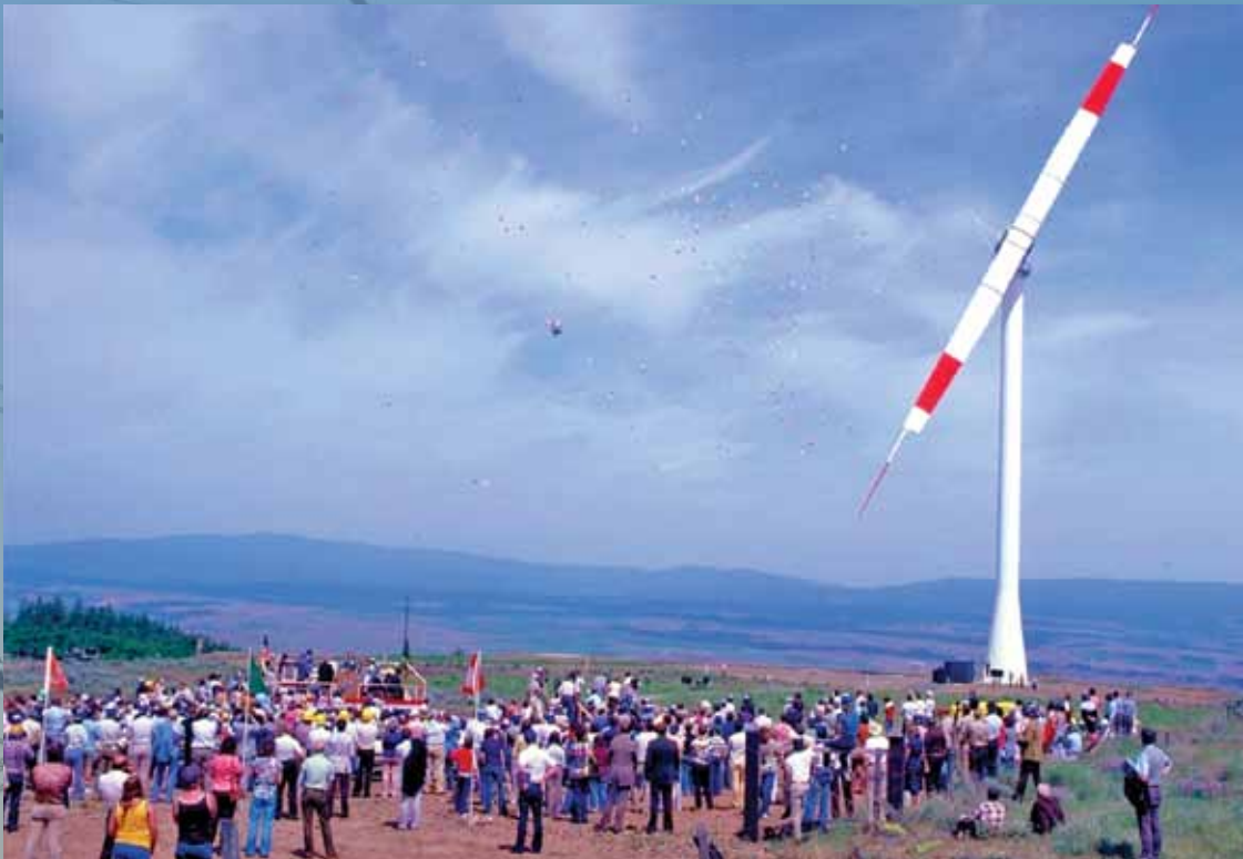
The MOD-2 wind project in south central Washington was dedicated into service May 1981. Commercial-scale operation began about a year later and continued over the next five years under this pioneering test project.
