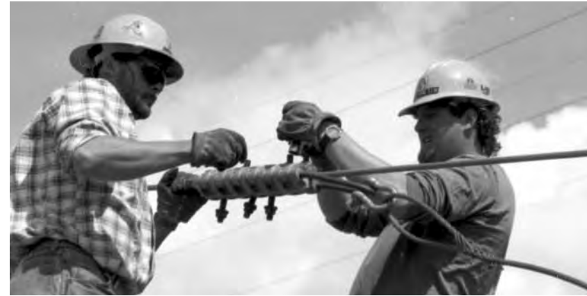
BPA crews have installed thousands of miles of fiber optic cable on existing transmission towers.
