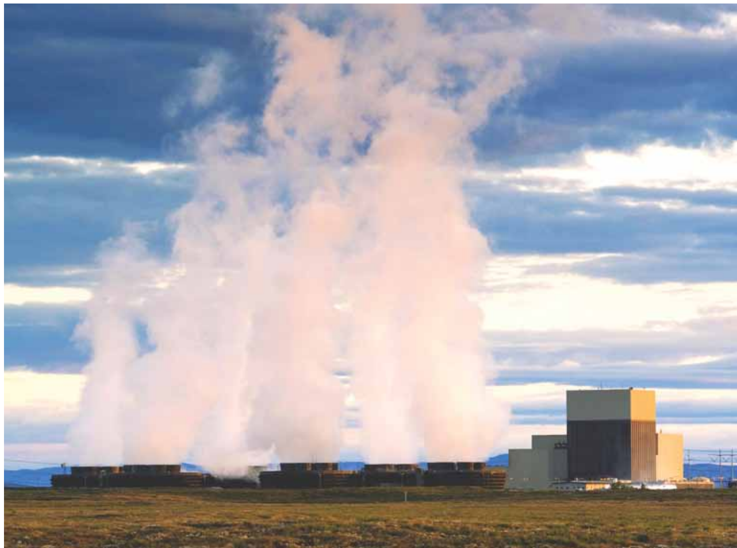
BPA funds and markets the power from the Columbia Generating Station, originally called WNP-2. The plant’s reliable and emission-free power complements the federal hydroelectric system.
