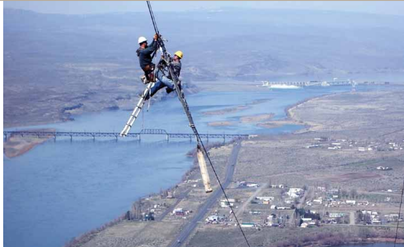
Far above the Columbia River, linemen install splice shunts on BPA's 230-kilovolt Midway-Vantage line. The shunts strengthen lines without taking them out of service, saving ratepayers millions of dollars. (Barry Peckham/BPA)
