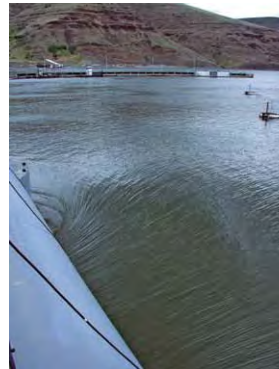
Water from the surface of the Snake River swirls over a spillway weir at Lower Granite Dam. (Scott Bettin/BPA)
