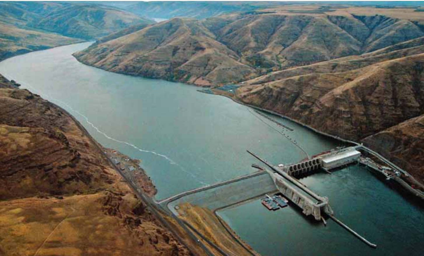
Lower Granite Dam on the Snake River. Some argued for breaching the earthen section of the dam on the left. (Idaho Statesman)
