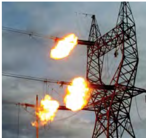
BPA used implosive fittings during construction of its Grand Coulee-Bell line. The fittings employ explosives to compress a metal sleeve around the end of the conductor, locking it into place.
