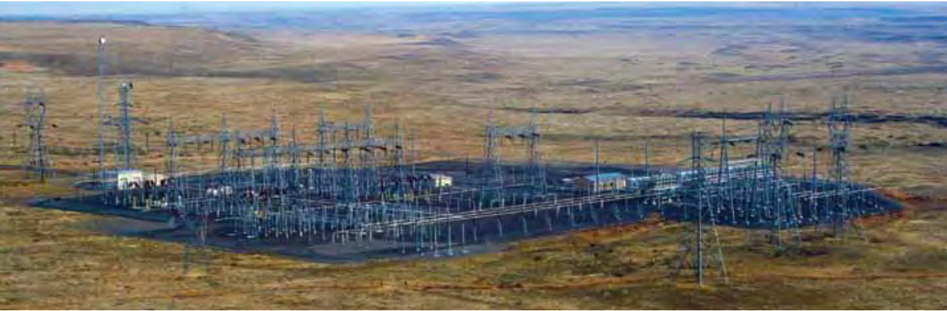
In the heart of the Columbia River Basin's wheat-growing region, BPA's Slatt Substation became home to the world's first 500-kV flexible alternating-current transmission system devices, or FACTS, which control the flow of power on transmission lines.
