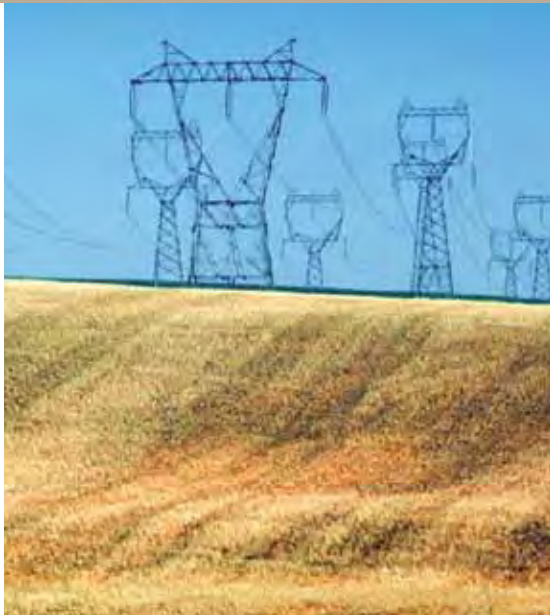
The first two AC intertie lines were constructed in the 1960s as an electric highway between the Northwest and Southwest.
