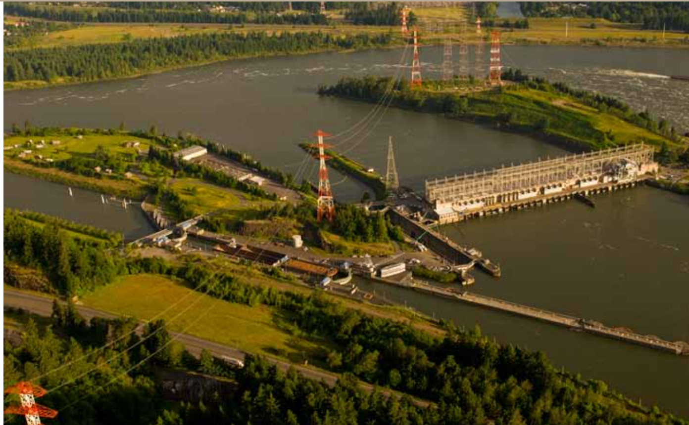
The U.S. Army Corps of Engineers completed a rehabilitation of Bonneville Dam’s first powerhouse in 2010, installing turbine runners that are safer for fish and rehabilitating power generation equipment that had been in service for nearly 70 years.
