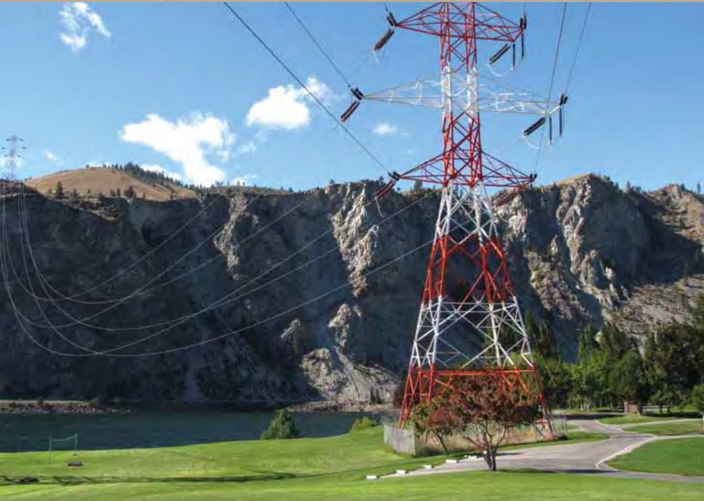
Red and white paint on transmission towers near airports or flight paths makes them more visible to pilots. The Federal Aviation Administration switched its requirements to lights on tall towers, but BPA maintains paint on towers marked under the older protocol. (Mitchell Brown/BPA)
