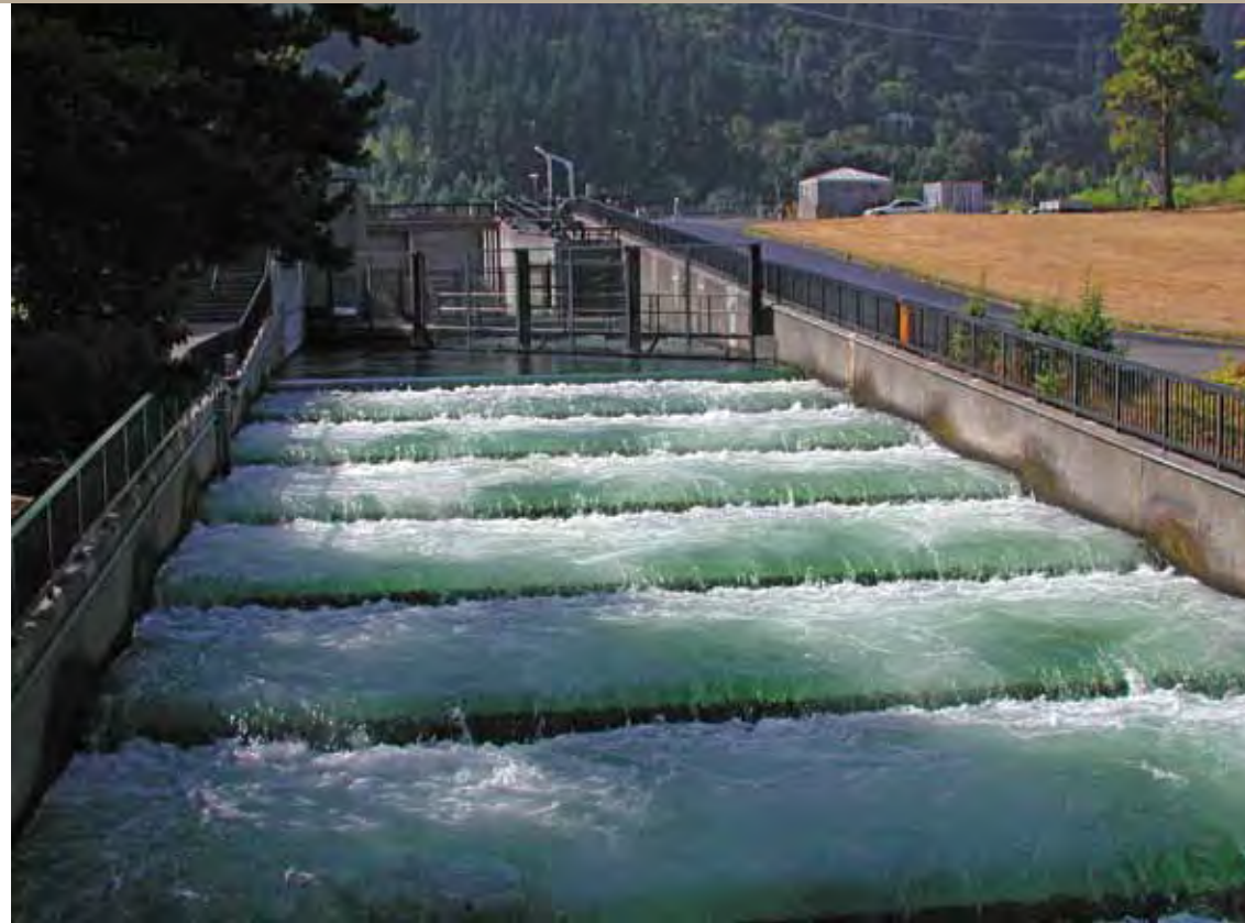
Fish ladder at Bonneville Dam.
