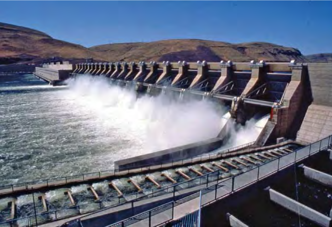
John Day Dam has the greatest generating capacity — 2,160 megawatts — of the four federal dams on the lower Columbia River.
