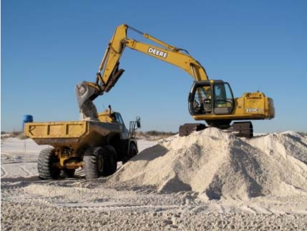
Figure 10. "Operation Deep Clean" excavation activity near Gulf Shores, Alabama, 8 January 2011.
