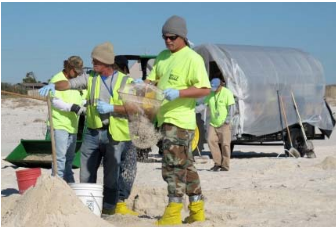
Figure 13. Manual cleanup of buried oil at Bon Secour National Wildlife Reserve, Alabama, 8 January 2011, showing the hand-sieving of oiled sand to remove oiled material.
