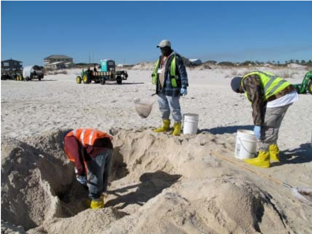
Figure 12. Manual cleanup of buried oil at Bon Secour National Wildlife Reserve, Alabama, 8 January 2011. Workers are unearthing a buried lens of oil for removal by hand-sieving.
