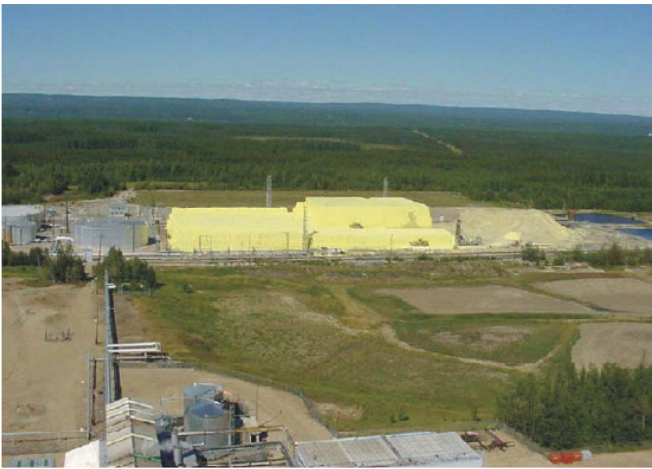
Figure 2. Elemental sulfur accumulating as a result of acid gas processing at the Zama Gas Plant in Alberta, Canada. As part of NETL's Regional Carbon Sequestration Partnership (RCSP) Validation Phase effort, the Zama Gas Plant is capturing and sequestering a co-contaminant stream of carbon dioxide and hydrogen sulfide (H 2 S) for enhanced oil production purposes. Co-sequestration reduces the accumulation of and treatment costs for elemental sulfur for the Zama Gas Plant. While not an electric generating facility, the RCSP Validation Phase efforts at the Zama Plant are a good example of co-sequestration capture and subsequent geologic storage.
