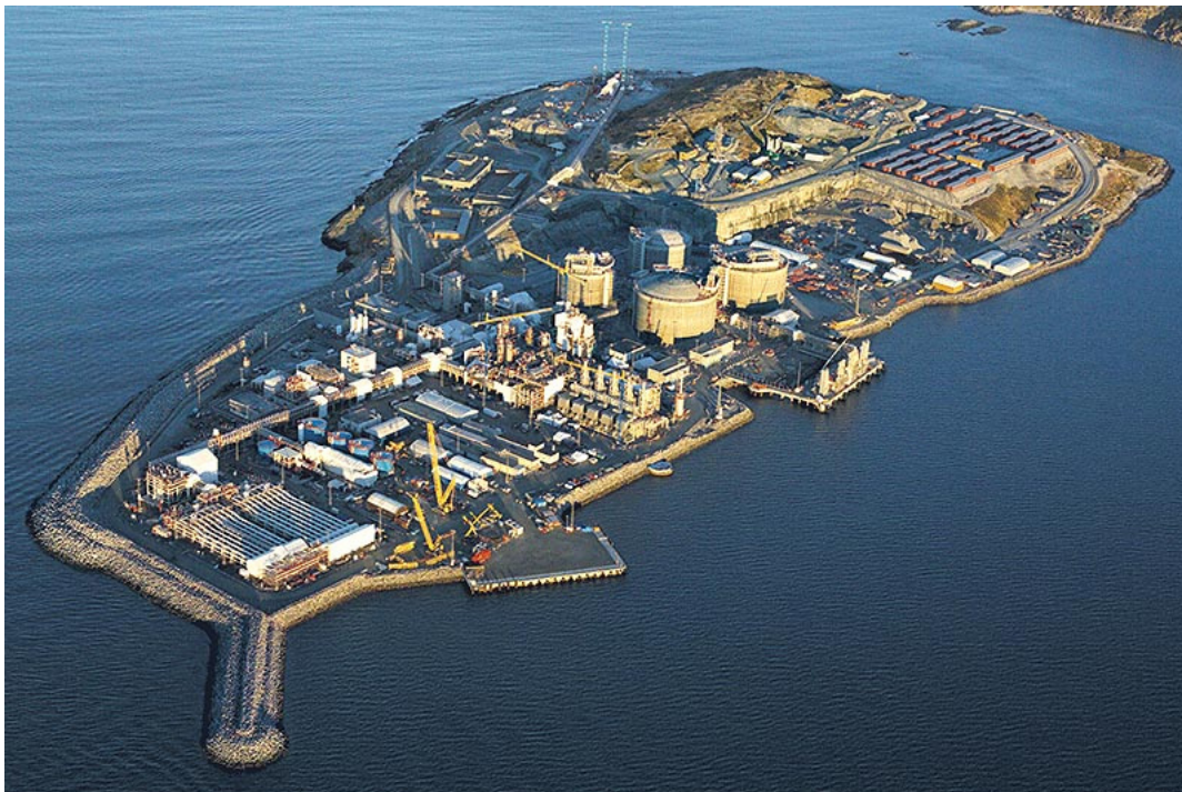
Figure 2: The liquefied natural gas plant at Melkøya, Norway (pictured) captures carbon dioxide from the production stream in sub-sea wells in the Barents Sea. CO 2 is separated and transported through a dedicated pipeline back to the sub-sea reservoir as part of the Snøhvit Project.
