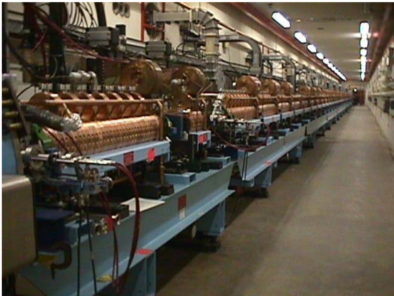
Figure B.2: Fermilab linac after upgrade in the tunnel.
