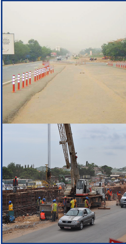
The N1 highway before construction, top, and during construction, bottom.
