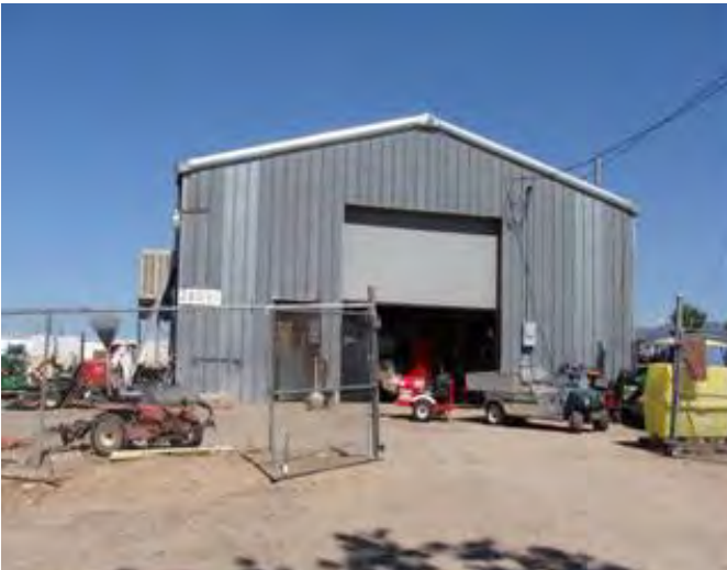
Maintenance complex provides minimal indoor storage.
