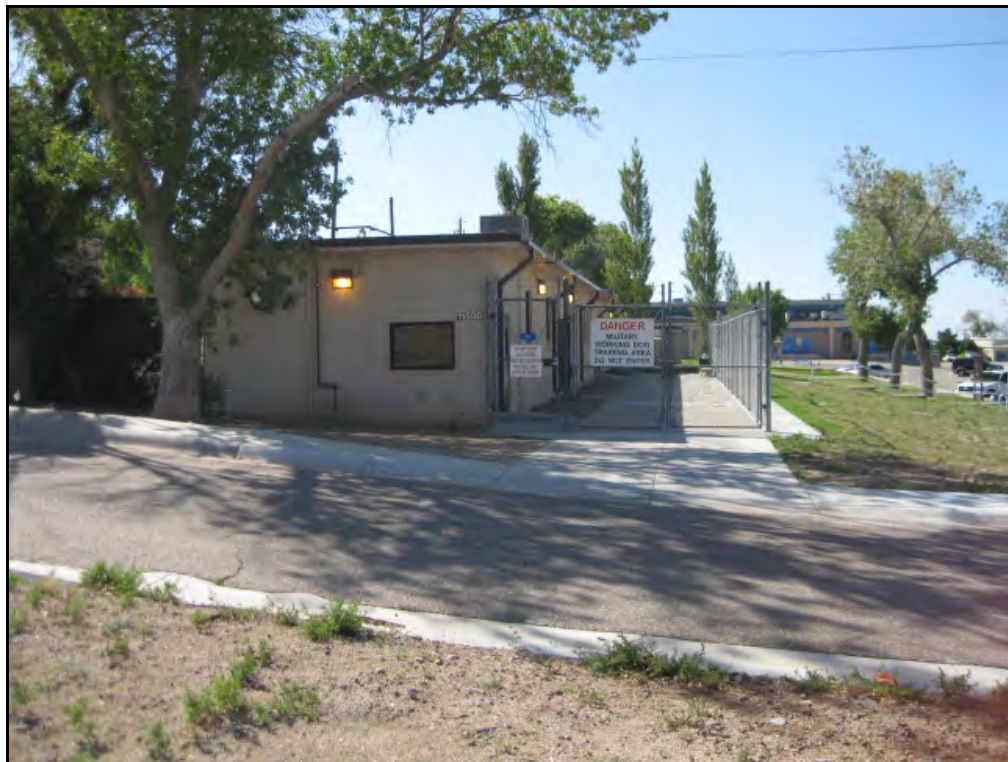
C2. Existing MWD Facility, Building 30126
