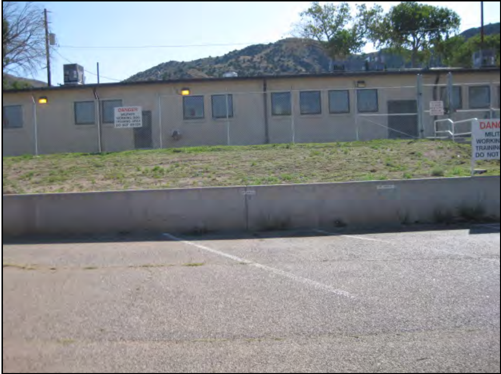
C1. Existing MWD Facility, Building 30126
