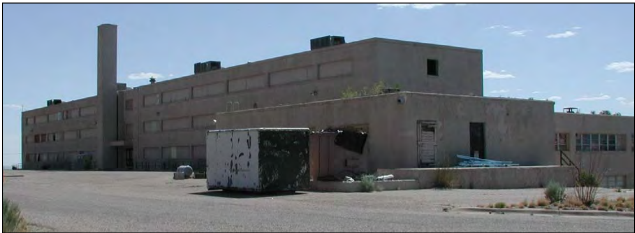
Figure 3-3. Current Visual Conditions at Four of the Buildings Proposed for Demolition
