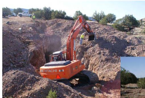
MD in the mine shaft was excavated and placed onto a specially-designed table for sorting.
