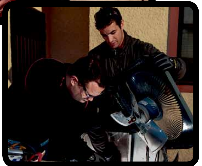
Tiago Rodrigues, 65th Civil Engineer Squadron HVAC Maintenance mechanic, checks the air pressure of the air conditioning external unit Feb. 22.
