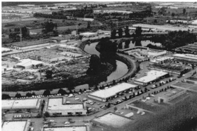
Figure 6-1. Regulated river with levees on meandering alignment
