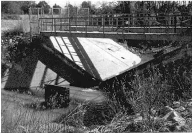
Figure 6-12. Flume-type grade control/gauging structure
