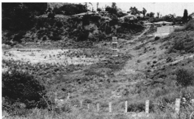
Figure 6-14. Debris basin and dam at head of alluvial fan
