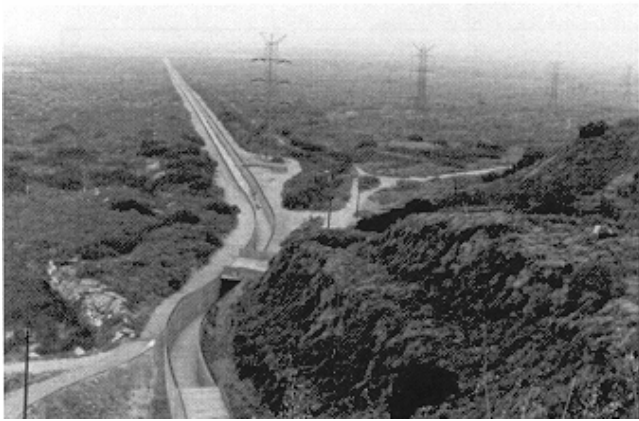
Figure 6-16. Concrete-lined channel on alluvial fan below debris dam (looking downstream)
