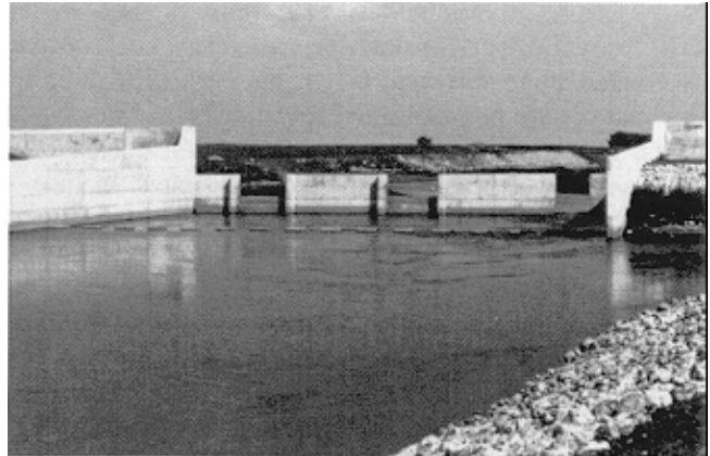
Figure 6-9. Use of stepped sill on grade control structure to match upstream rating curve
