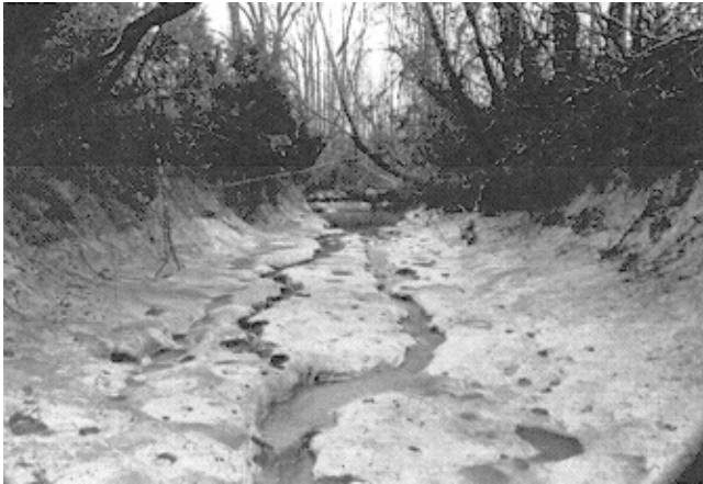
Figure 4-8. Nick zone in degrading channel (clay layer)
