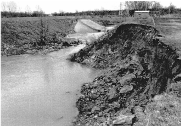
Figure 4-6. Bank failure
