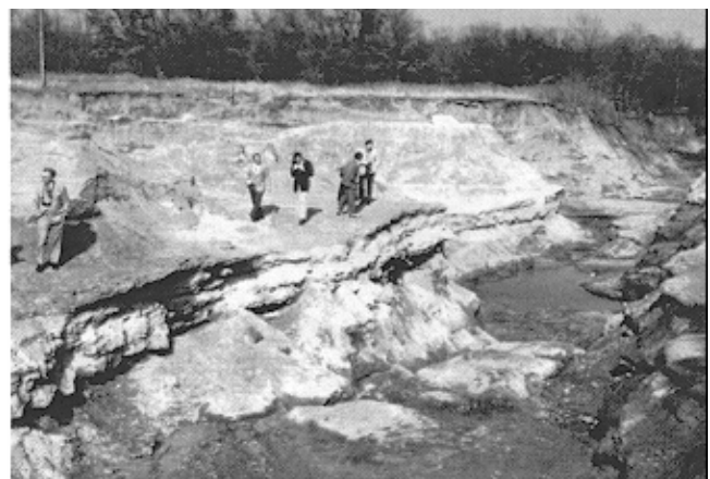
Figure 3-13. Grapevine Spillway Channel after erosional episode
