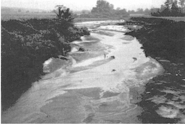
Figure 3-11. Induced instability upstream of channel enlargement, Twenty Mile Creek
