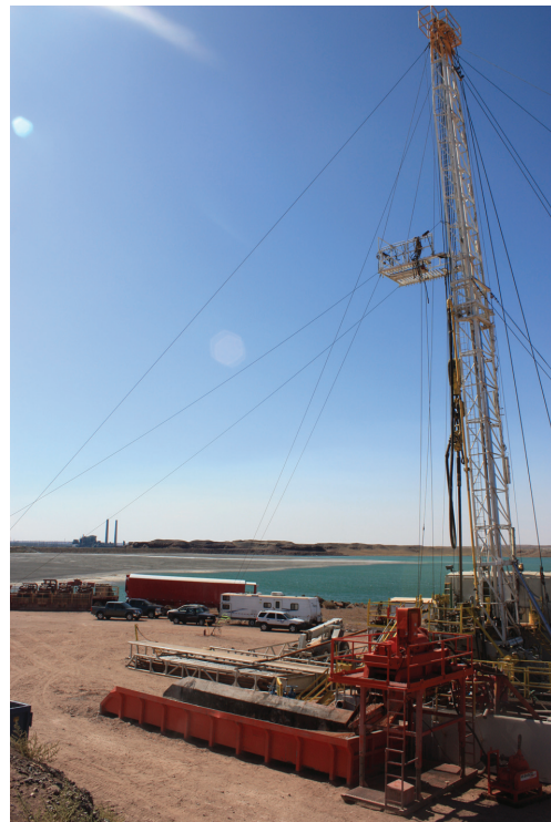
Figure 18. WESTCARB Test Drilling Site. (Courtesy of WESTCARB Website)
