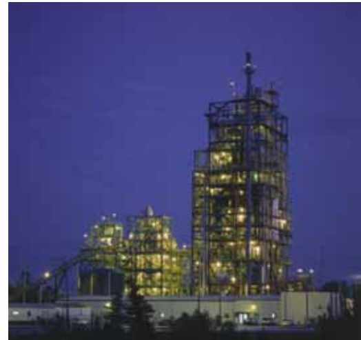
Power Systems Development Facility
