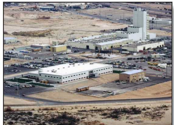
North Las Vegas Facility (source: NSTec Facility Data Warehouse, September 2006)
