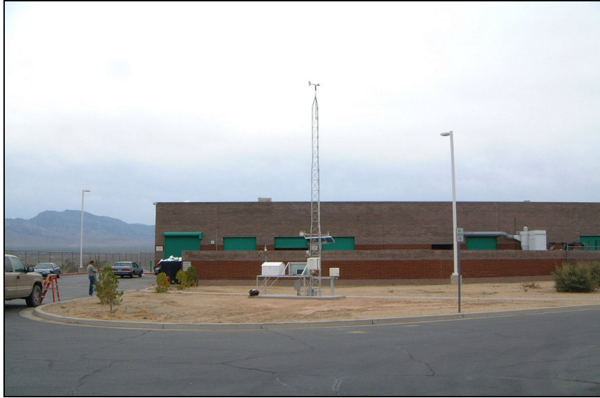
Figure 7-2. CEMP Station at Mesquite, Nevada
