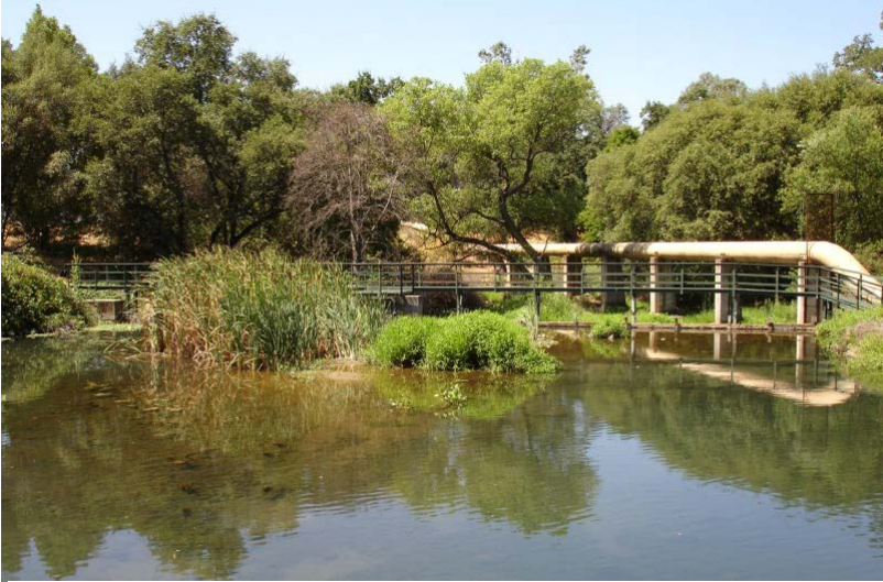
Looking downstream toward Asbury Diversion Dam and Asbury Pipeline. A new flow measurement weir will be installed at the dam to ensure a minimum of 5 cfs is released in Baldwin Creek.
