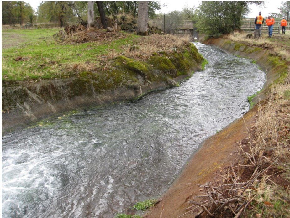
Looking downstream of Pacific Power Canal where a culvert crossing will be constructed to provide road access to the new fish barrier.
