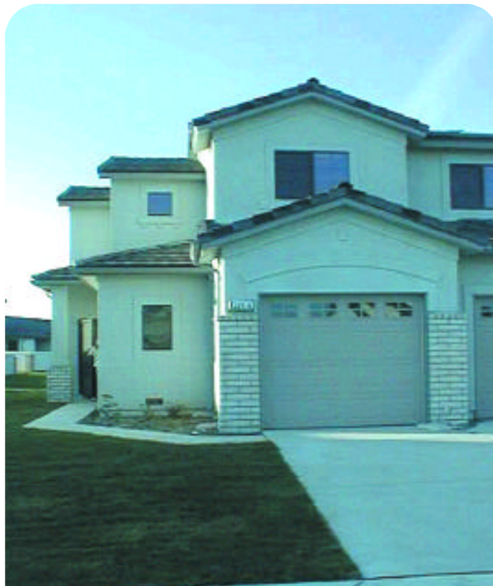
New Family Housing Unit at Naval Air Station, Lemoore, CA.
