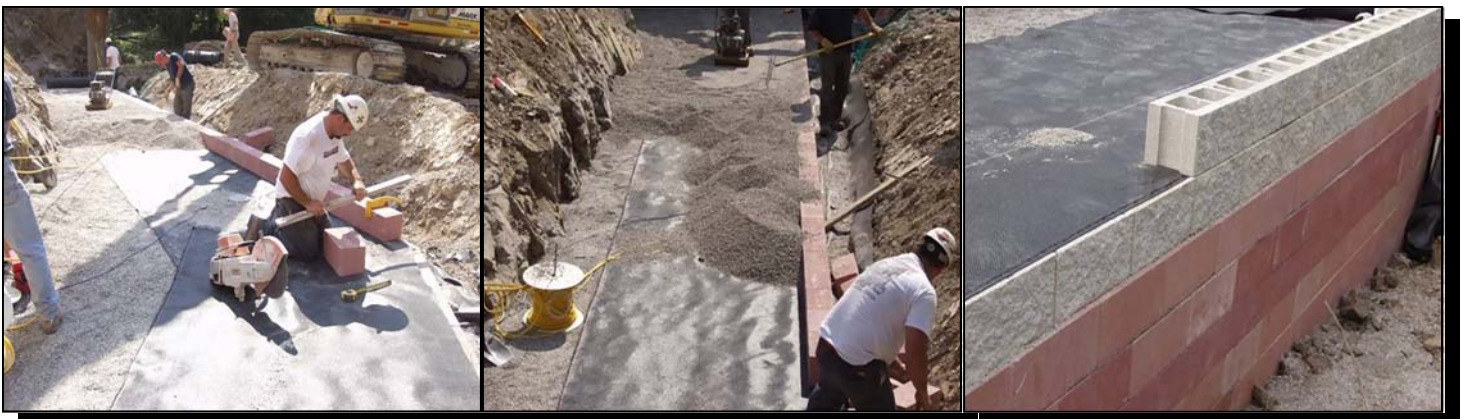
3. Add Layer of Geosynthetic Fabric (Reinforcement). Repeat until desired height is achieved.
