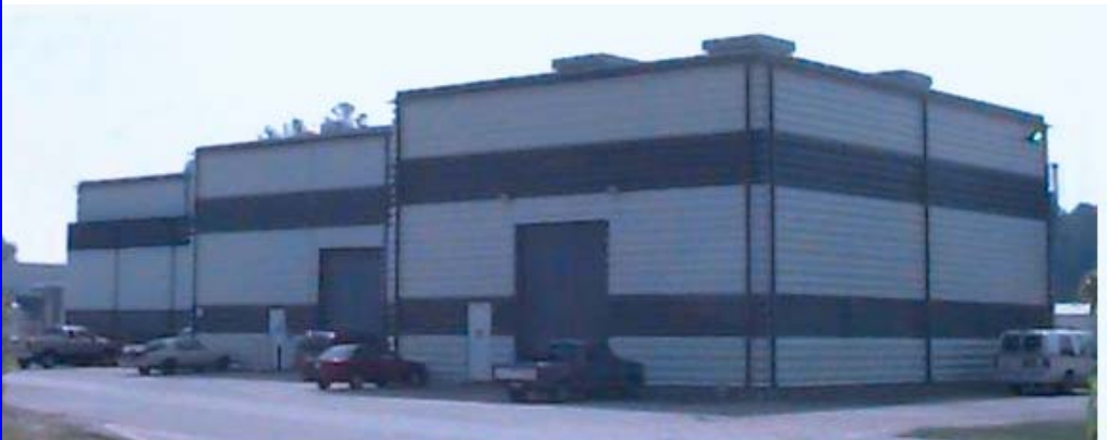
Central Helium Liquefier Complex
