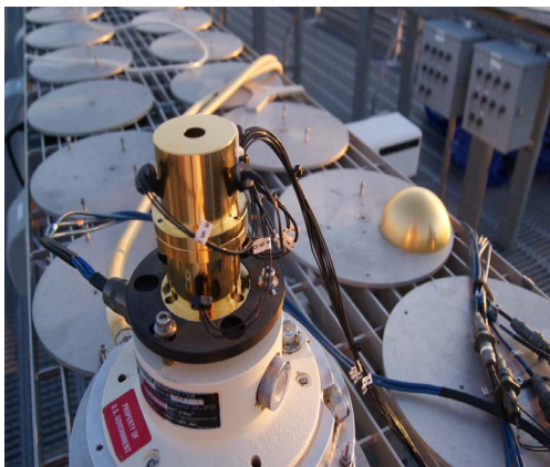
Fig. 1. ACP outdoor set-up at NREL/SRRL
