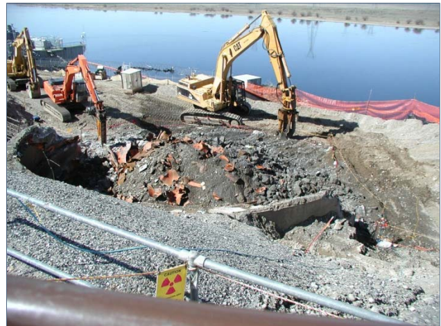
Removing concrete debris and piping from the River Corridor
