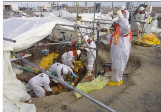
Removal of Transfer line in Tank Farms
