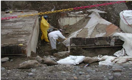
Removal of Waste Container from Burial Ground in the Central Plateau
