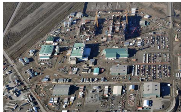
Construction of the Waste Treatment and Immobilization Plant
