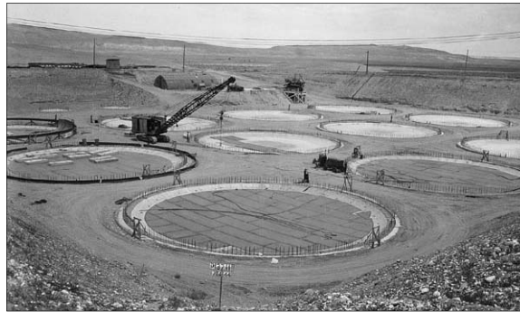
Construction of Hanford Tank Farm
