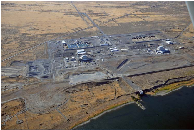
K East and K West Reactors
