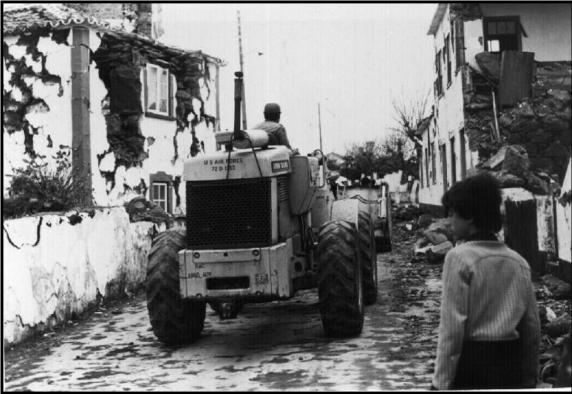
An Air Force bulldozer clears rubble from a road after the 1 January 1980 earthquake.
