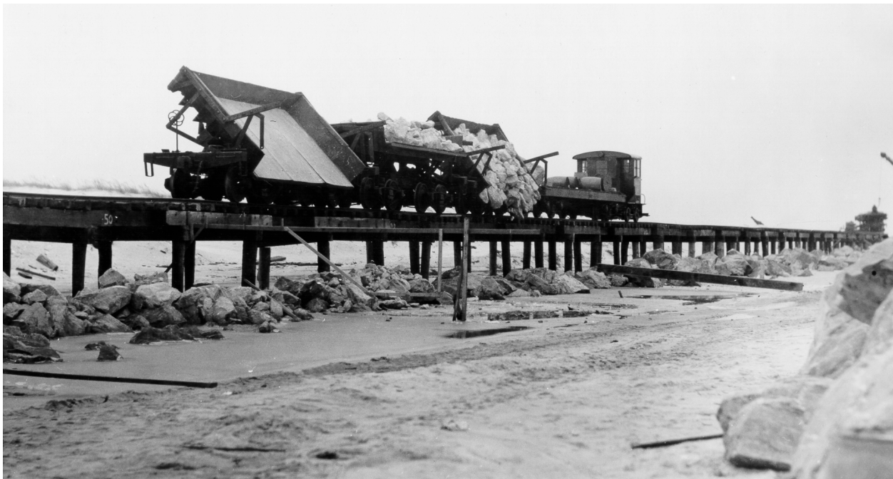
Figure I-3-6. Construction of Fire Island jetty on Democrat Point, at the west end of Fire Island, Long Island, New York. Many early USACE jetties were built from the land moving seaward using materials brought in by train. Photograph taken 3 Jan 1940, from Beach Erosion Board Archives.
