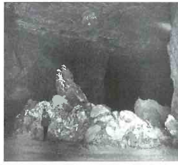
Figure 2 - Large roof fall at underground limestone mine.
