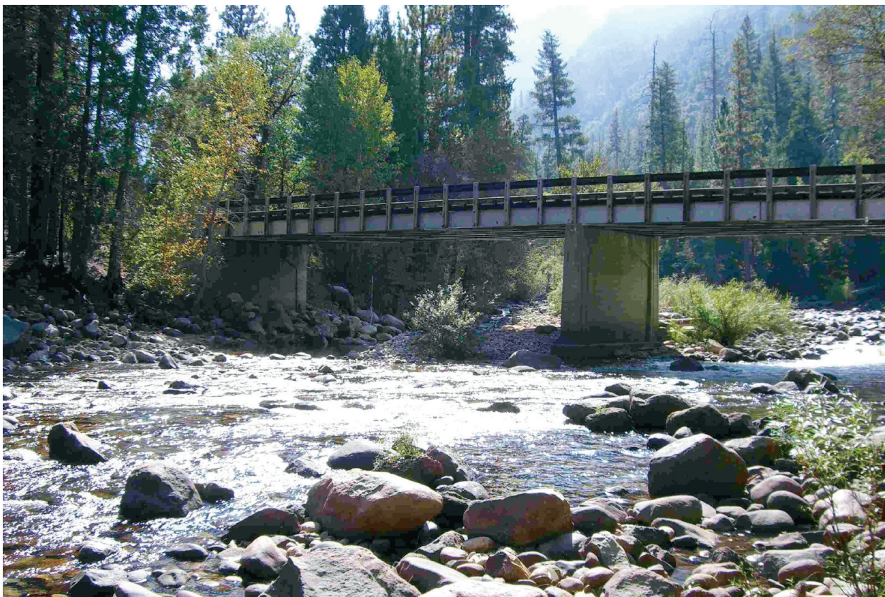
Cedar Grove Village Bridge, Kings Canyon National Park (Smillie, 2007).
