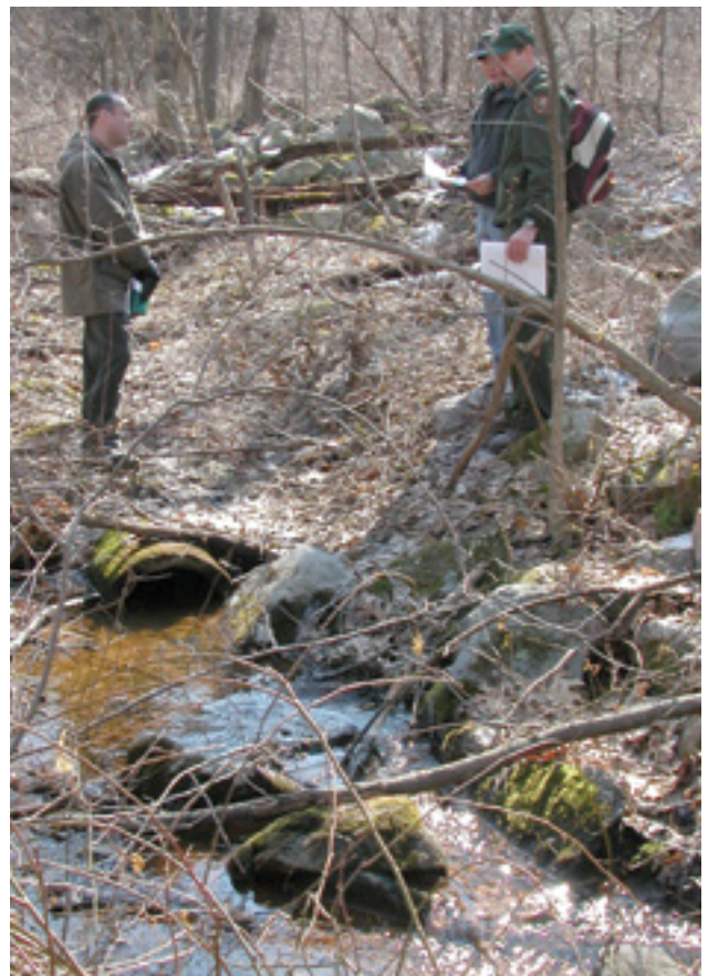
Concrete outfall before restoration (NPS, 2003).
