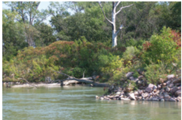
A small gap in bank revetment on the Missouri River allows increased habitat values (NPS 2006).
