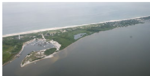
Above: Aerial view of Watch Hill Marina from the bay side of Fire Island.
