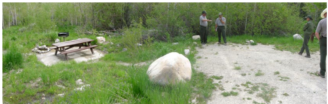
A campground parking space on the fill. Note the concrete pad and table also in the wetland with groundwater exposed in the firepit. Great Basin National Park (Nevada). NPS/K. NOON
