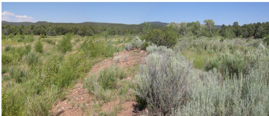
A manufactured levee (center) separates recently restored riparian/wetland habitat (left) from Glorieta Creek (right, hidden by vegetation). The levee constrains natural biological and hydrologic processes in the riparian corridor and is a potential source of excess sediment deposition into nearby aquatic systems. Pecos National Historical Park (New Mexico). NPS/JOEL WAGNER
