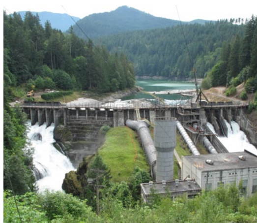
Elwha Dam from downstream with Lake Aldwell impounded in the background, taken from the webcam on 24 August 2011. Olympic National Park (Washington). NPS COLLECTION
