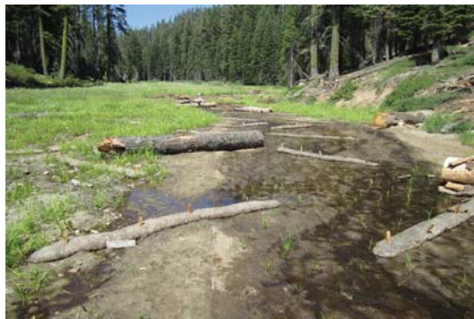
Repair/treatment of the erosion channel, funded (in part) by this money
