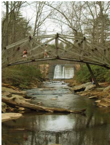
Crescent Bridge, Prince William Forest Park. (NPS Photo)
