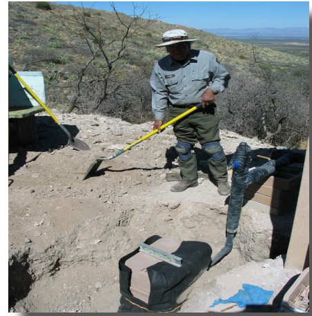
Installing new flow meter at Fort Bowie National Historic Site (Reber, 2008)
