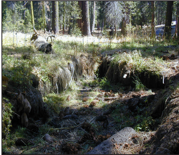
Sunset Meadow headcut before restoration (Demetry, 2008).
