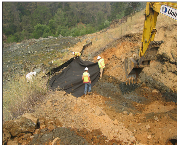
Photos left to right: Pucinella Project - Caltrans engineers installing a road underdrain above Spring 1 (E. Wolf, 2008); Measuring Pucinella growth (NPS, 2008).
