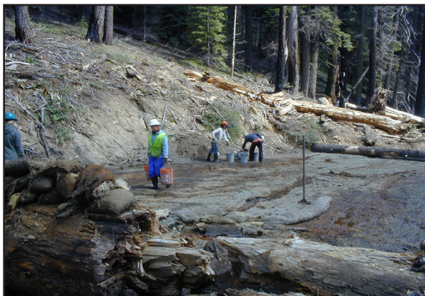
International volunteers moving fill material for minor erosion repair at Upper Halstead Meadow, Sequoia National Park (Demetry, May 2008).
