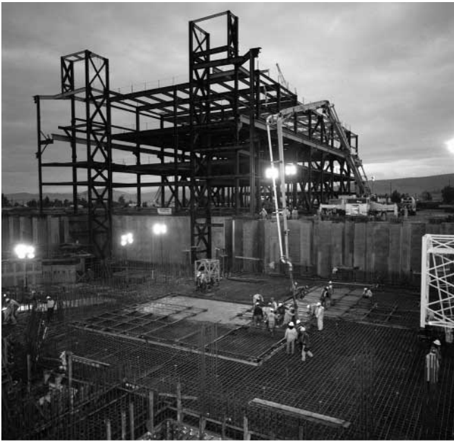
FIGURE 1. Switchyard 1 concrete pour. (40-60-0598-1213#7pb01)
