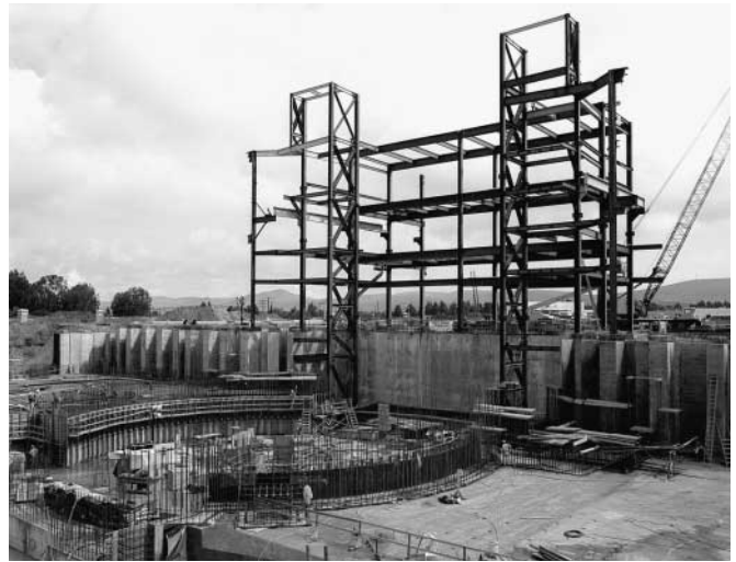
FIGURE 2. Looking north from Switchyard 1. (40-60-0598-1007#3pb02)
