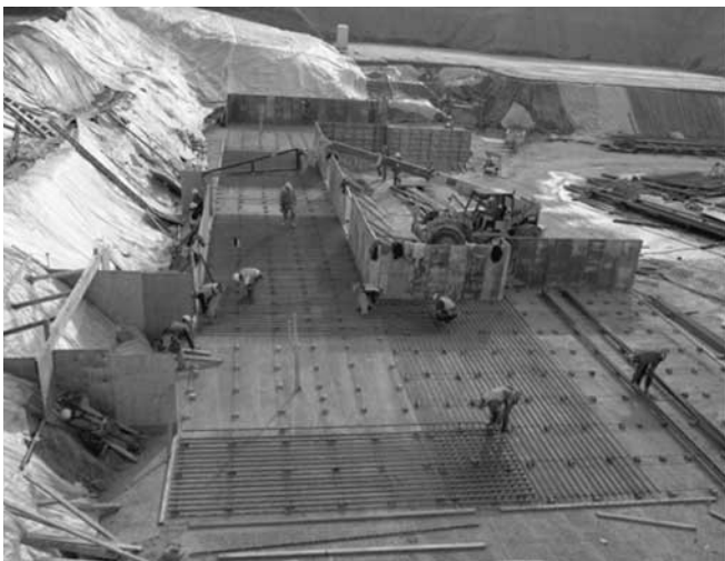
FIGURE 1. Target Bay footing construction. (40-60-1297-2604pb01)
