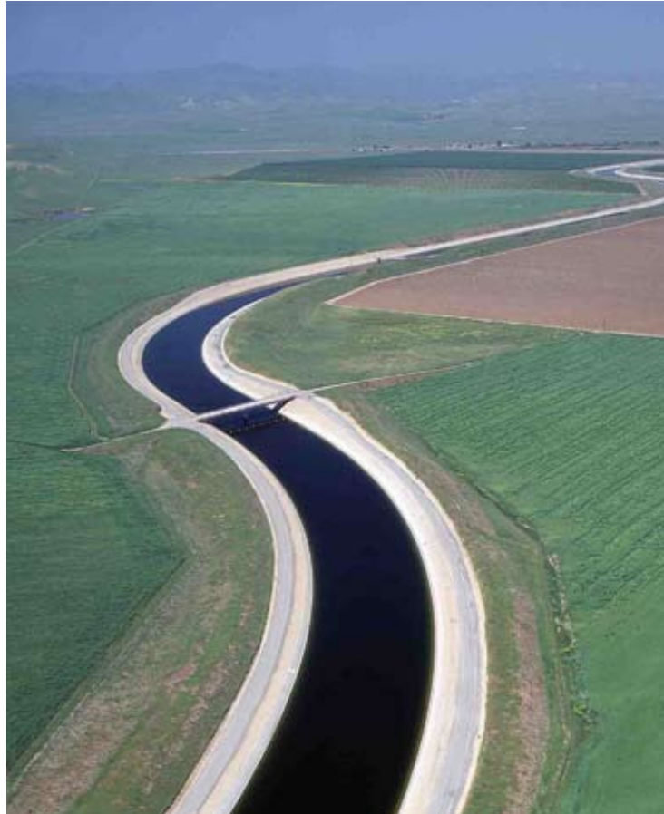
The California Aqueduct is a crucial part of that state’s infrastructure.
