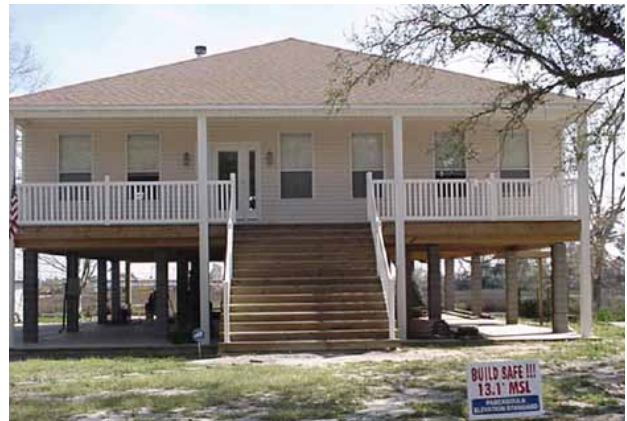
Elevating existing structures can help protect them from storm surge and other flood events.
