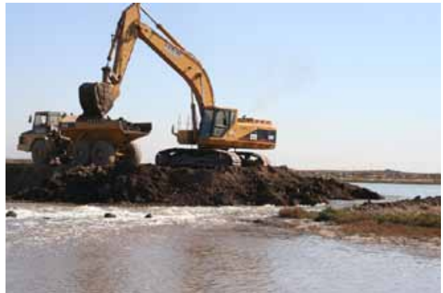
Removing or breaching manmade levees can be an effective way to restore natural processes.
