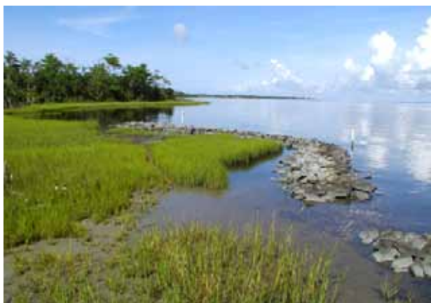
Hybrid shoreline stabilization structures that employ marsh plantings and low rock sills (to protect the vegetation) can help stabilize eroding banks.
