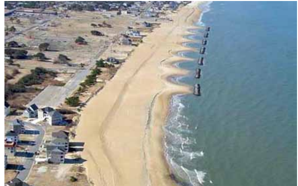
Offshore breakwaters can keep sand onshore, reducing the rate of shoreline erosion.
