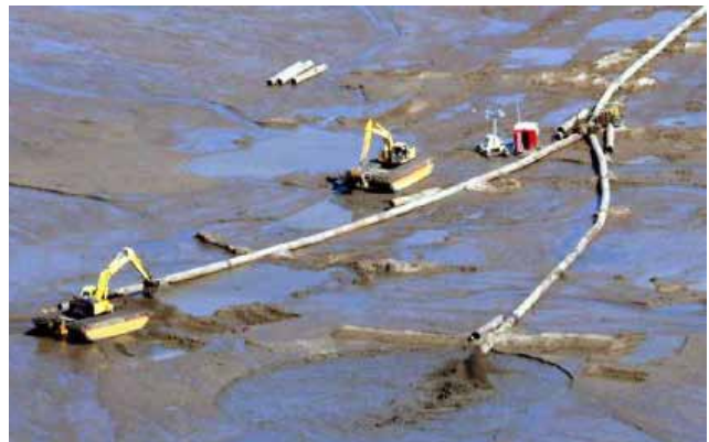
Sediment dredged from navigation and diversion channels can be used to restore and create wetlands.
