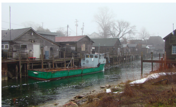
As Great Lakes water levels decline, ports and marinas will be increasingly ill-equipped to meet the needs of shipping and fishing vessels.
