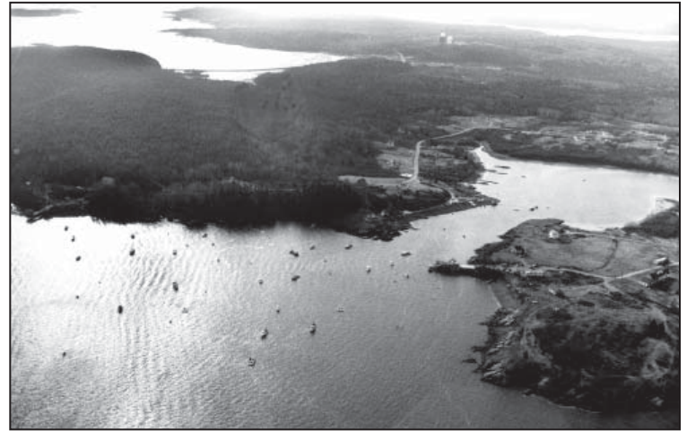
Aerial view of Bucks Harbor, which is located in Machiasport on Machias Bay, about 25 miles southwest of Eastport, Maine. (Click photo for high-resolution version)
