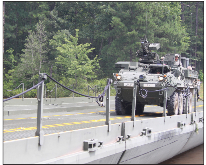
Soldiers from the Pennsylvania Guard's 56th Stryker Brigade Combat Team conduct a tactical water crossing July 24 over a 120-meter long bridge constructed by the Bowling Green-based 189th Multirole Bridge Company, 276th Engineer Battalion, 91st Troop Command at White's Lake on Fort A. P. Hill.
