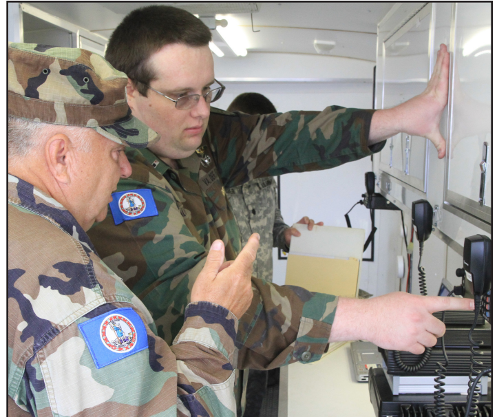
Members of the Virginia Defense Force conduct function checks on communications equipment in a Mobile Command Post trailer April 28 at Fort Pickett.
