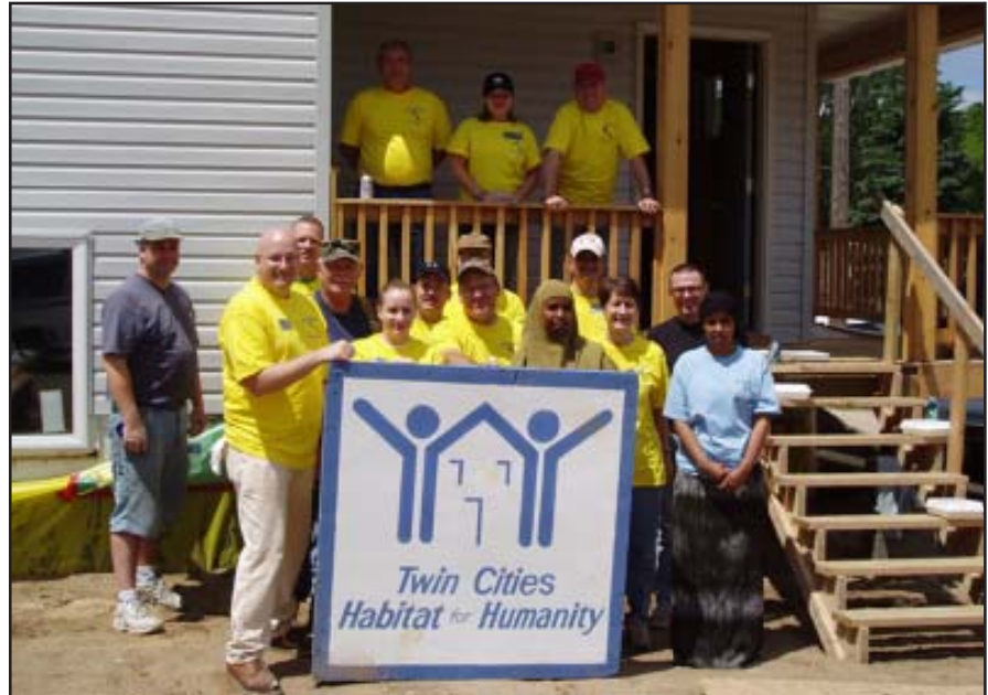
Members of the base services squadron help to construct the home of Khadra Hassan, a North Country Lodge employee.
