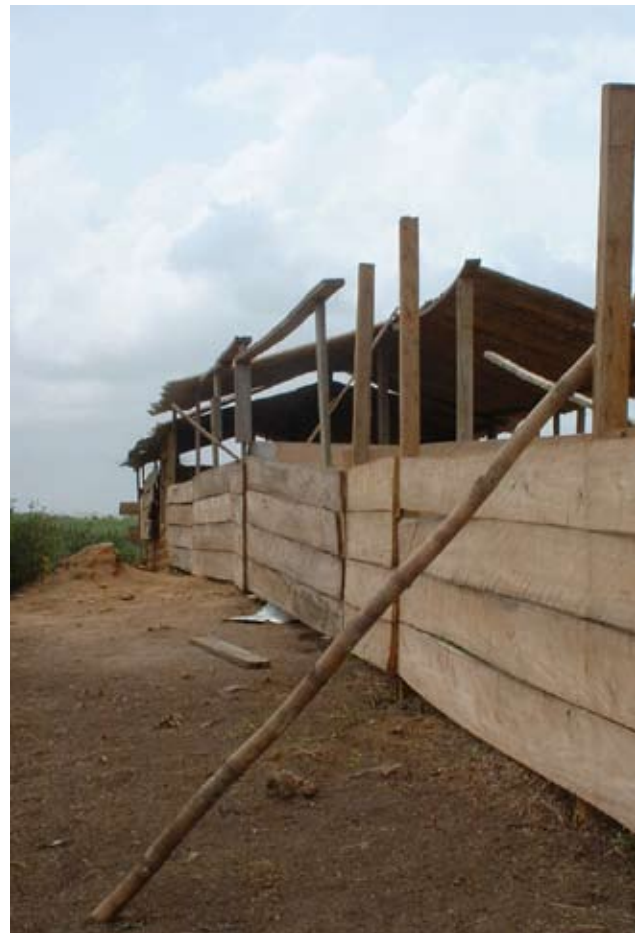
Above: Deforestation exposed this area to strong windstorms, destroying the new corrugated roof of the community school and toppling the walls. This inadequate replacement structure is intended to be temporary, but may be in service for many years.
