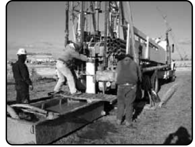
Rotasonic Drilling - The team used this method at OU 3. It is effective in areas with a lot of rubble, concrete, and debris.
